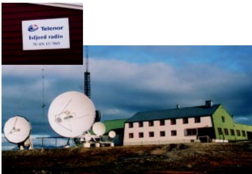
The main antenna is shown in the centre of the picture and on the left side, the spare antenna. Over the roof you catch a glimpse of the link antenna pointing towards the Svalsat station.
